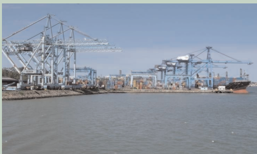
Post-Panamax cranes to unload/load container ships
